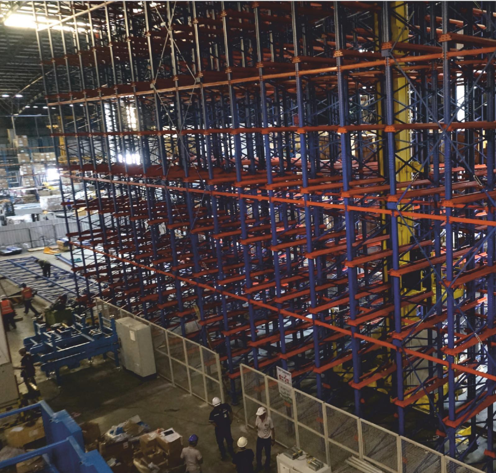
One of the busiest Air-cargo complexes in this region was looking for solutions for intermediate storage of cargo in cages. The ASRS was provided by the principal partners from Europe & the racking system was designed & produced in India. Supplied, Installed & commissioned by Jay Storage Solutions, this project was designed & executed with the local Seismic considerations & the fast paced environment of an Air-cargo complex.
